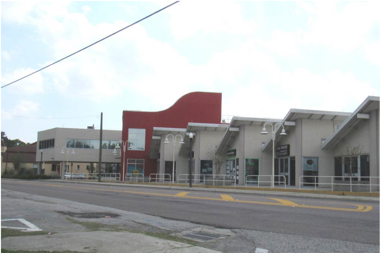
Existing development across Moncrief Road.
